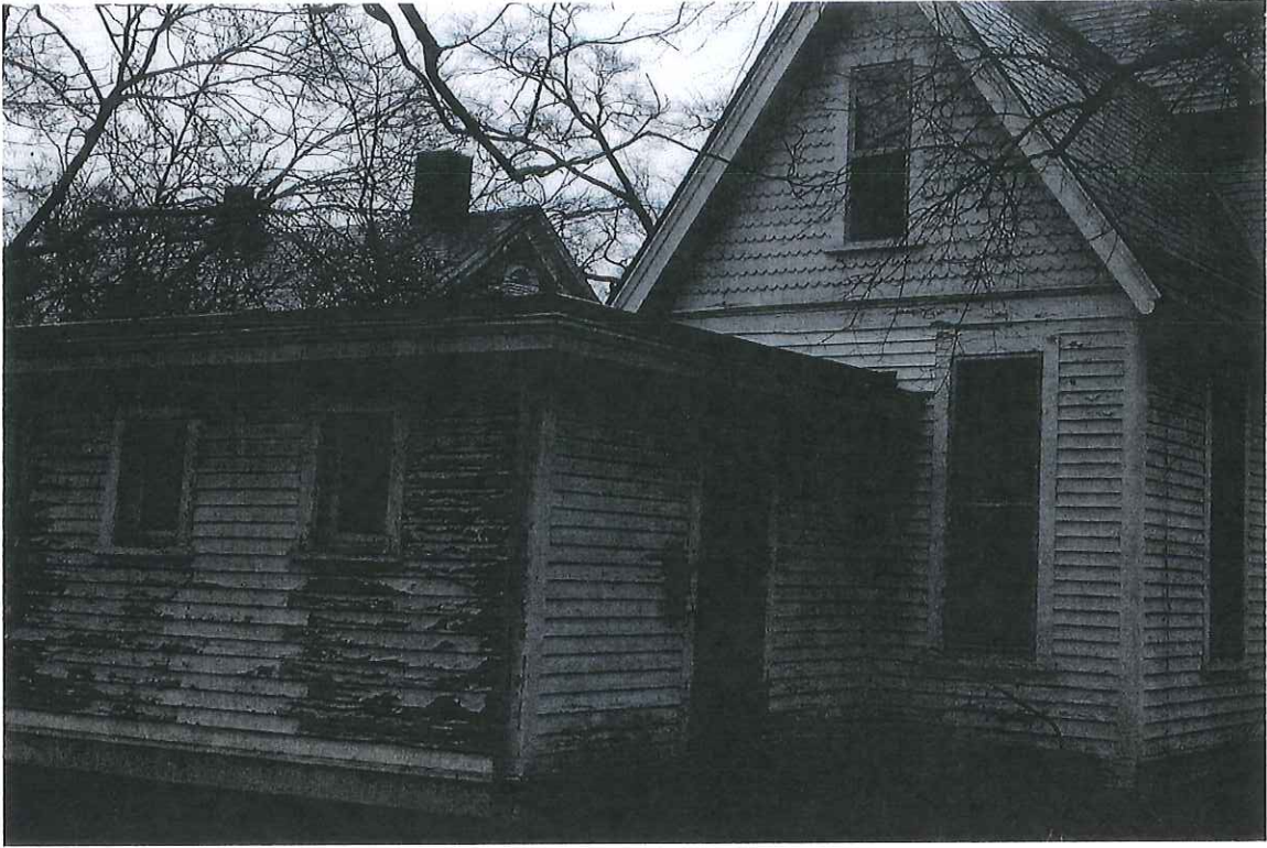
401 N. PERSON ST FROM SOUTHWEST REAR ADDITION WITH EXISTING DOOR
