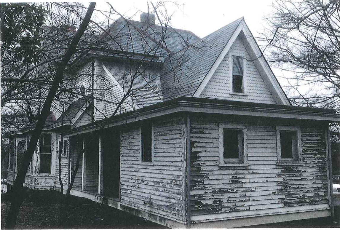
401 N. PERSON ST. FROM NORTHWEST EXISTING CONDITIONS
